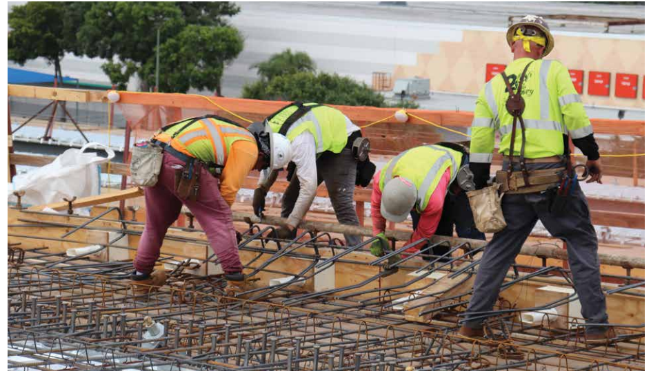
A crew from Shelby Erectors construct a new span of bridge.
